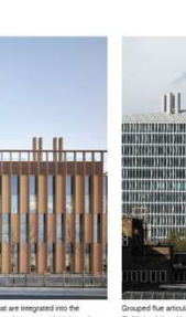
3.7.6 Flues integrated with the architectural strategy - primary facade material. Grouped flue articulation St Michael Uten Hub, London. Allies and Morrison
