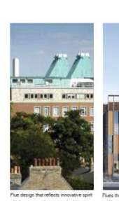
3.7.6 Flues integrated with the architectural strategy with high quality architectural expression. Anglia Ruskin University, Cambridge. Richard Murphy Architects
